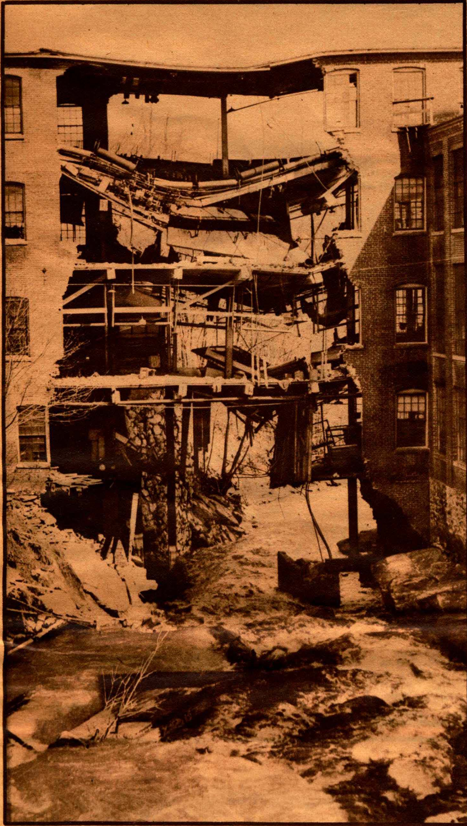
THE BLACKSTONE RIVER smashing through to the valley of Southern Massachusetts and into Rhode Island carried out four floors of this mill in the Cherry Valley section of Worcester.
