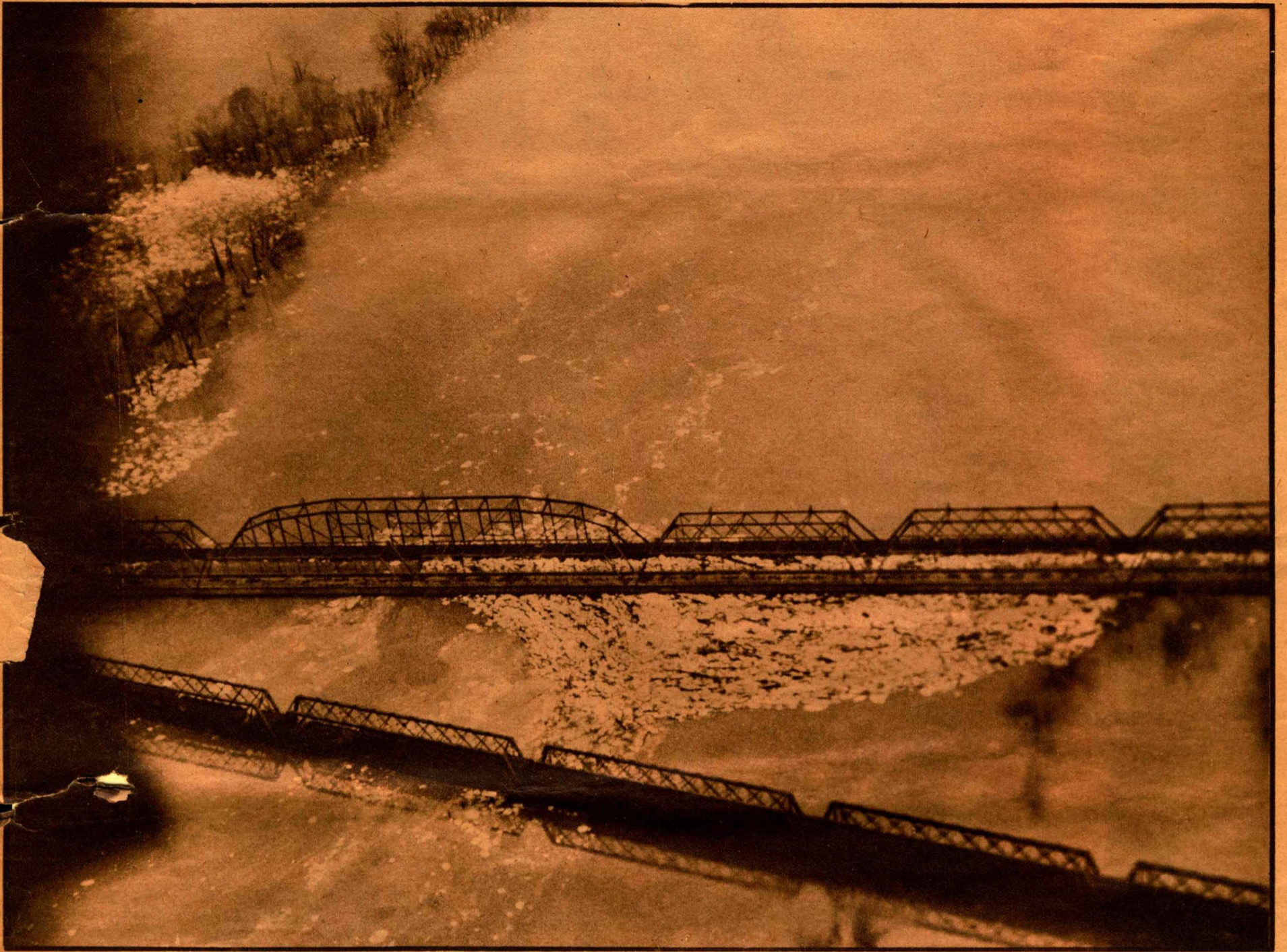
NORTHAMPTON-HADLEY bridges, clogged and wrenched by ice jams and surge, still span the Connecticut.
