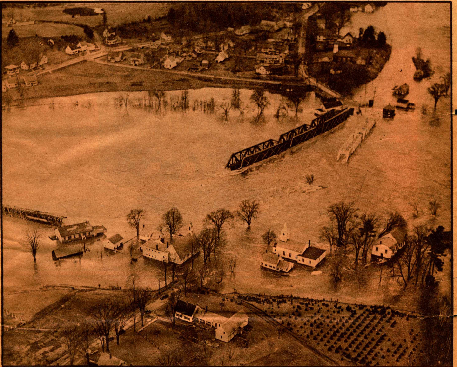
OUT of the mountain torrents and landslides came the floods to sweep away New Hampshire's bridges as these at Suncook on the Merrimac were lost. Globe photo by Edmund Bond
