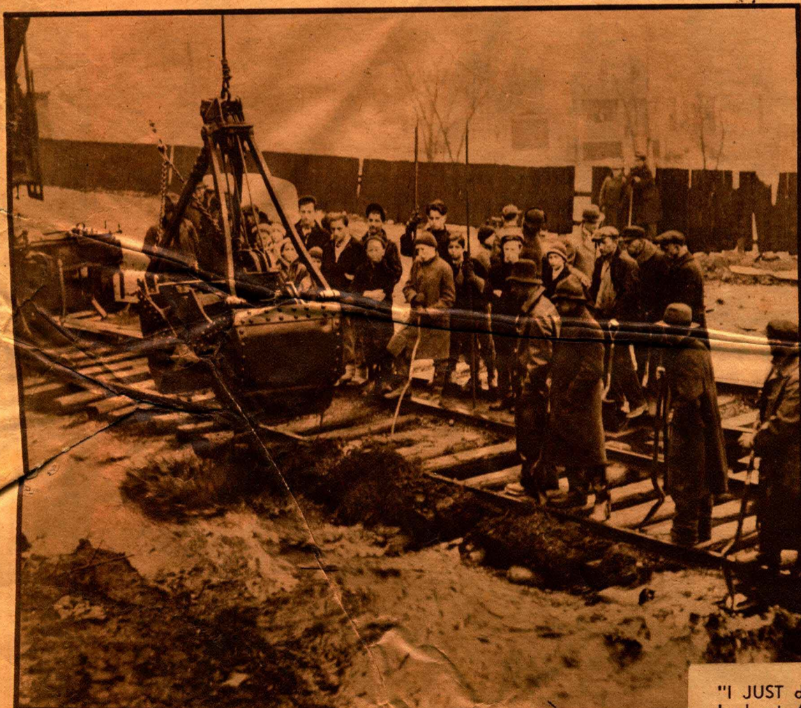
WRECKING CREW rebuilds the Boston and Maine through Arlington after flood washout. Globe photo, Paul Maguire.
