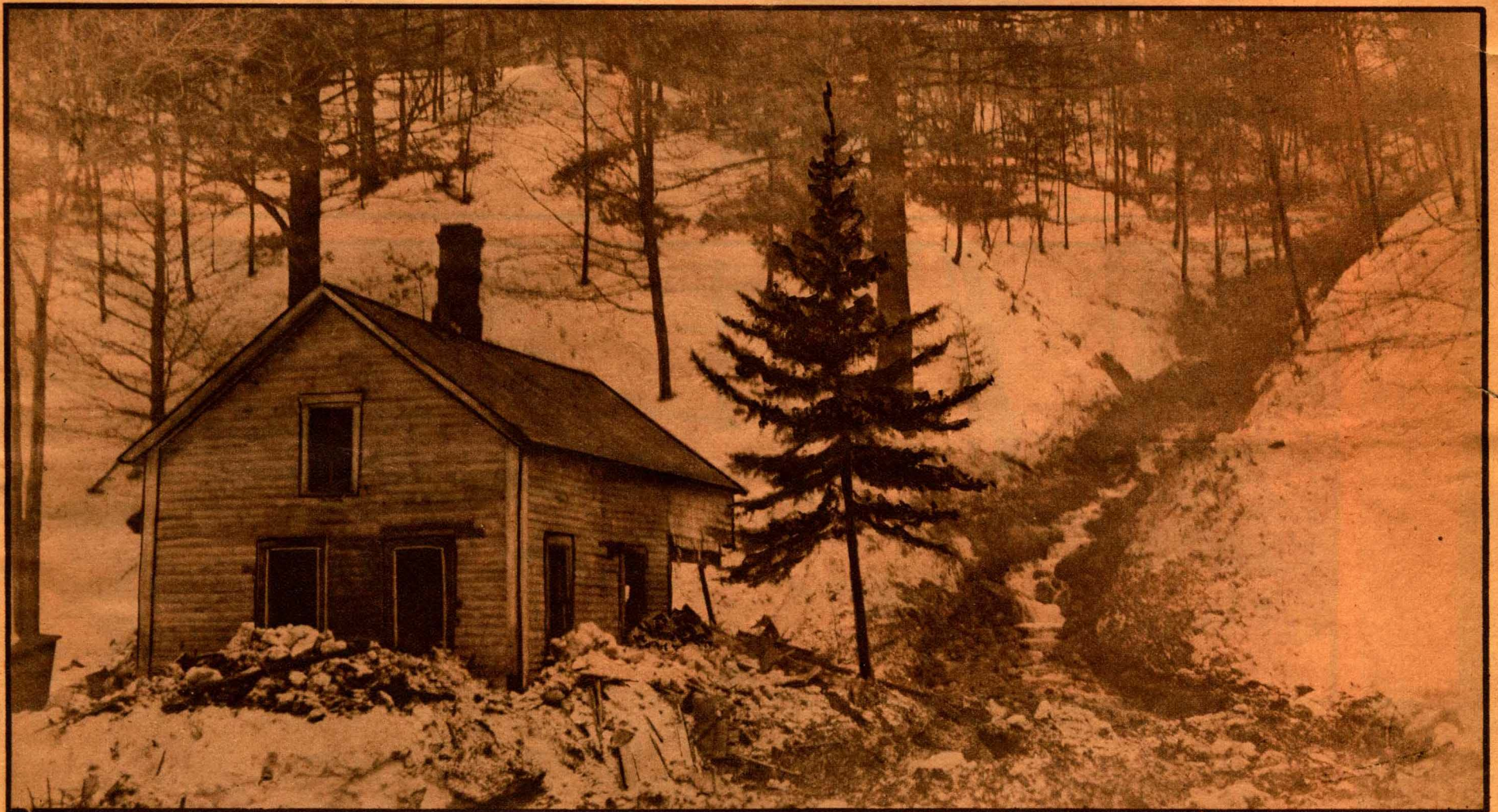
FIRST DEATH of the 1936 floods occurred in this house at Lower Bartlett in the foothills of North Moat Mountain, N. H. Eugene Hill was killed as an avalanche of snow and a torrent of water roared down to signal the beginnings of a flood that was to sweep to the sea. Belcher photo
