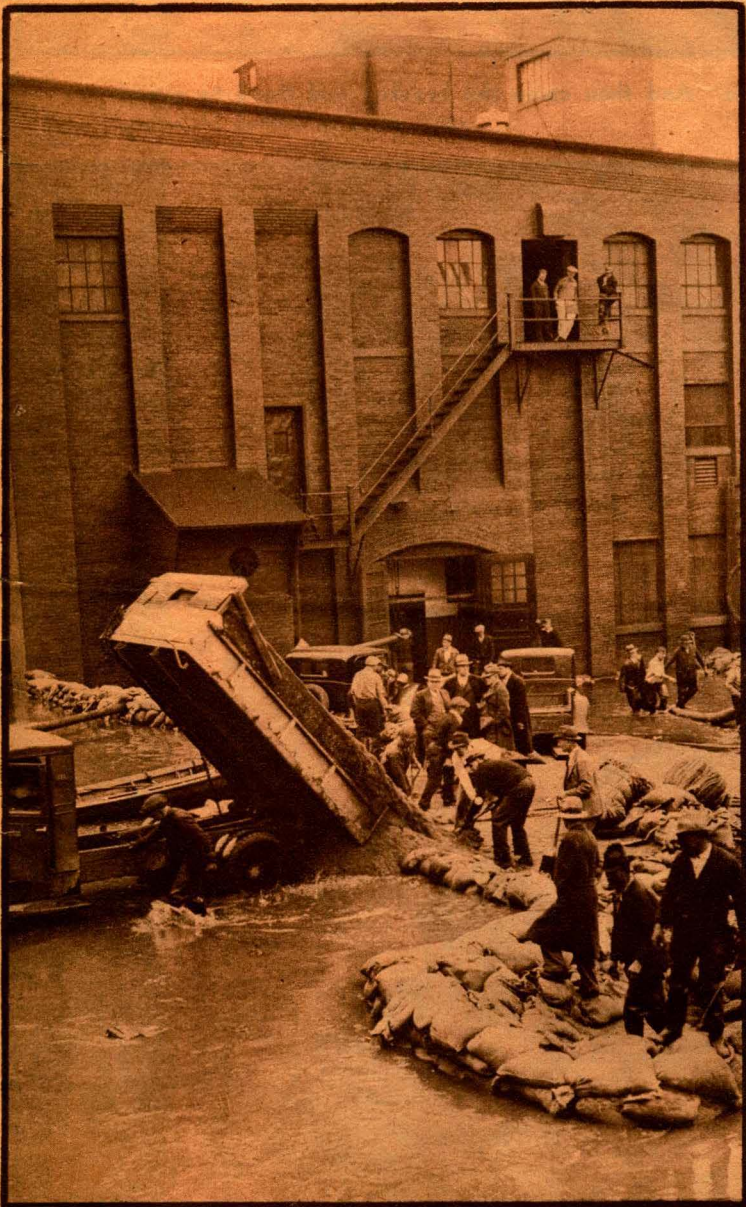
A DAM to save power in the Springfield Gas Company. It failed of its purpose as the river swept over the sandbags and shut off fuel for cooking to thousands. Globe photo by John Kelly
