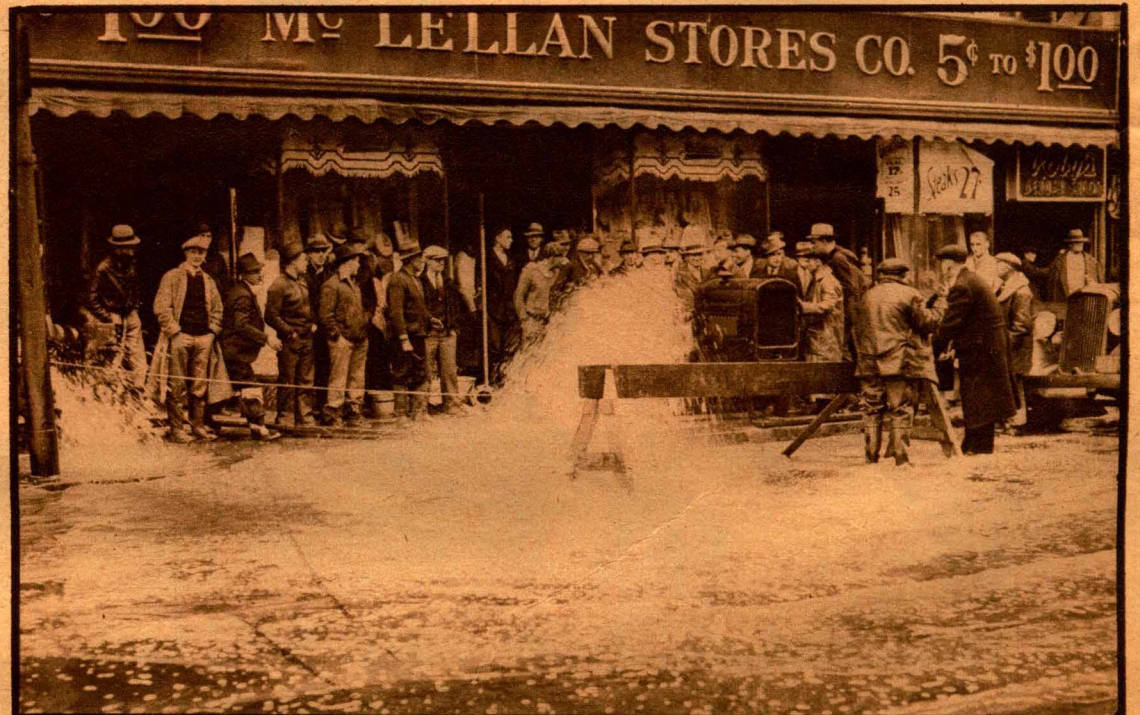
PUMPING OUT after the flood and deluge, in Springfield.
