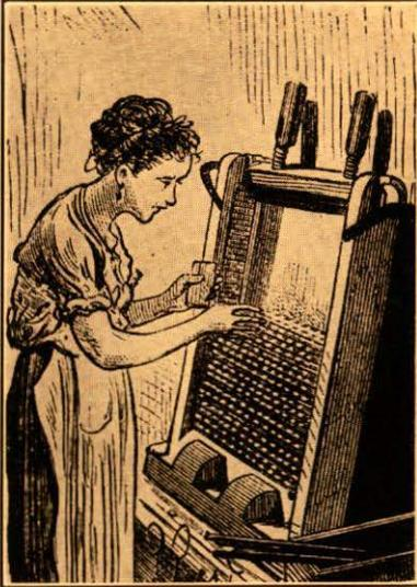
*Placing Matches in a Frame for Dipping*
