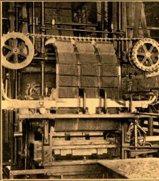
Cutting and Setting Matches in Plates of Automatic Match Machines
