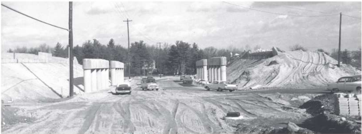
Rt. 110 looking toward Stedman Street Rt. 495 overpass under construction, 1959
