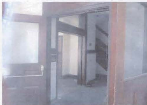
A View of the Inside of MCTS
