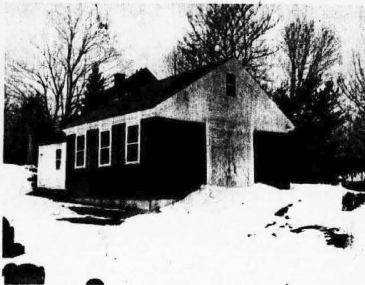
OLDEST SCHOOLHOUSE in town is subject of Article 61 on Town Meeting warrant. Frequently referred to as "the Hearse House," it was built in 1802 at easterly end of Forefathers Cemetery -- at a cost of $500. (Photos by George A. Parkhurst)
