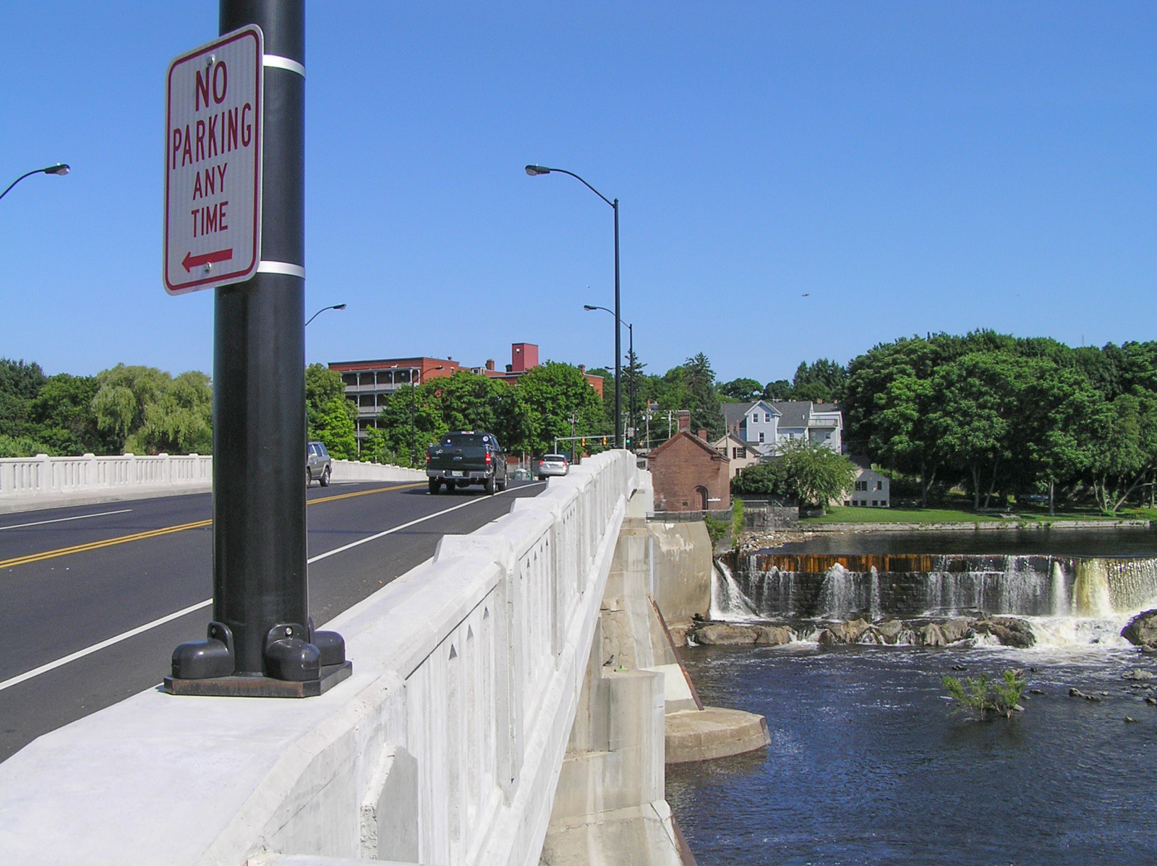
Newly completed roadbed on O'Donnell Bridge
