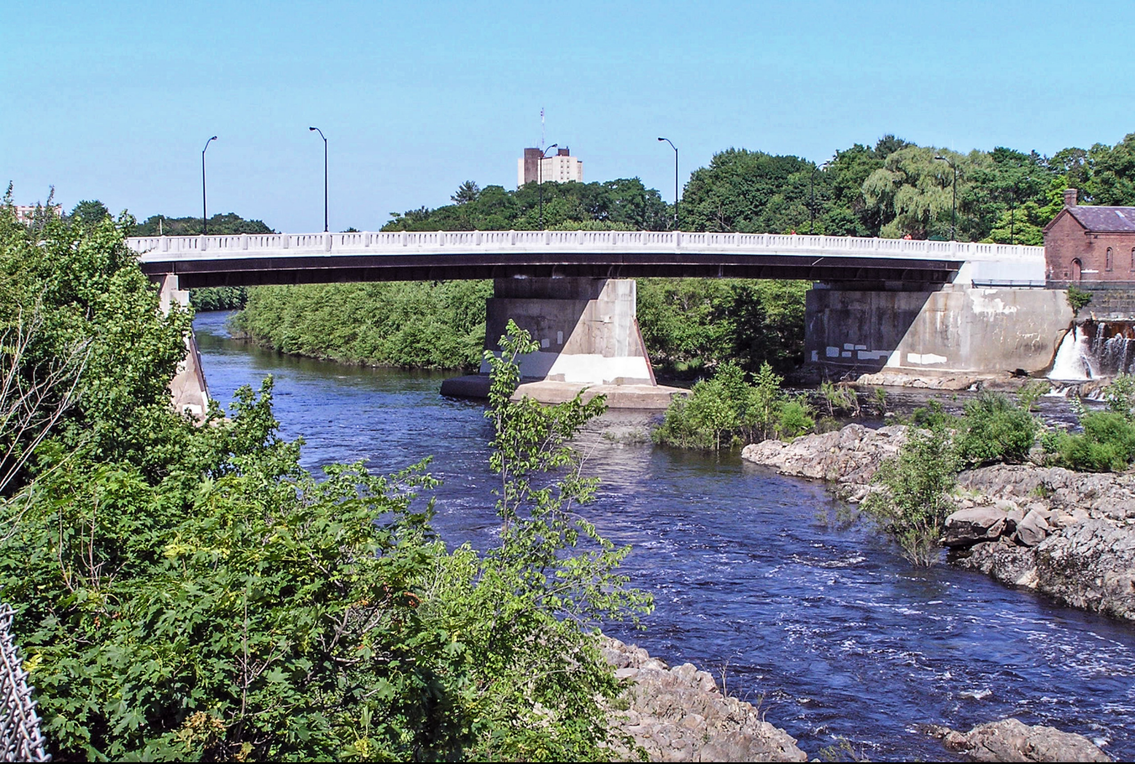
O'Donnell Bridge after reconstruction
