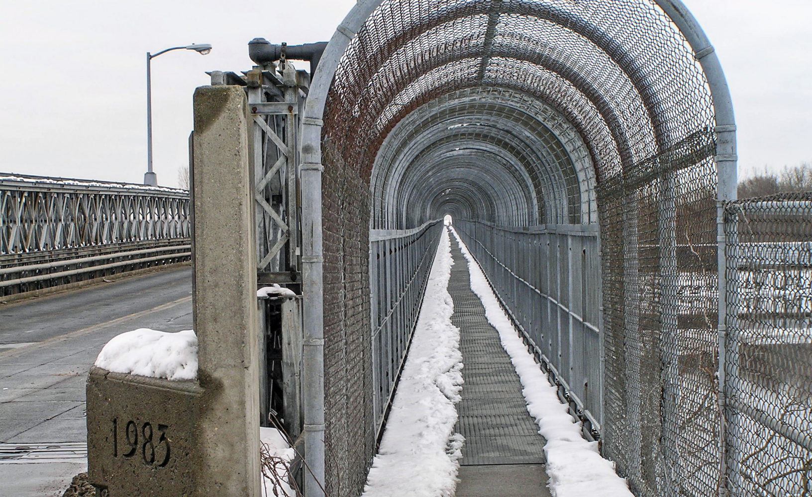
Rourke Bridge pedestrian passage
