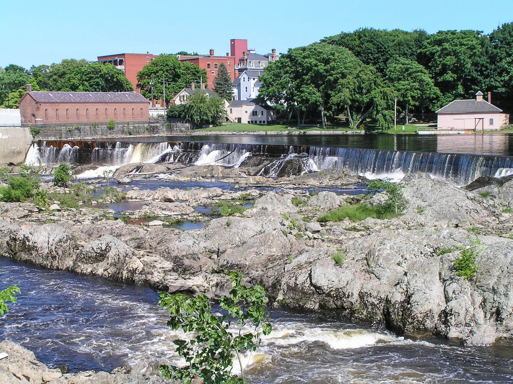
Northern Canal gate house and Pawtucket Dam blacksmith shop
