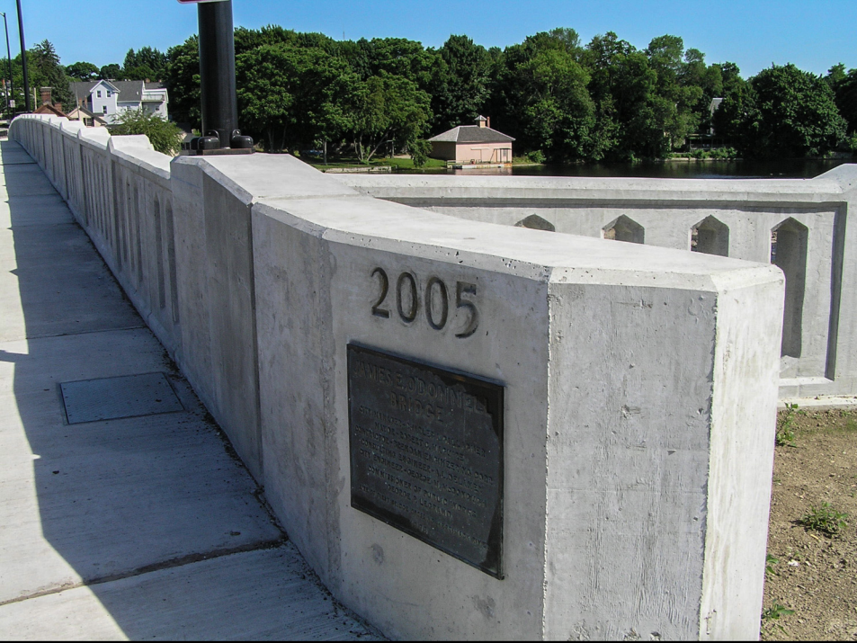
O'Donnell Bridge after reconstruction
