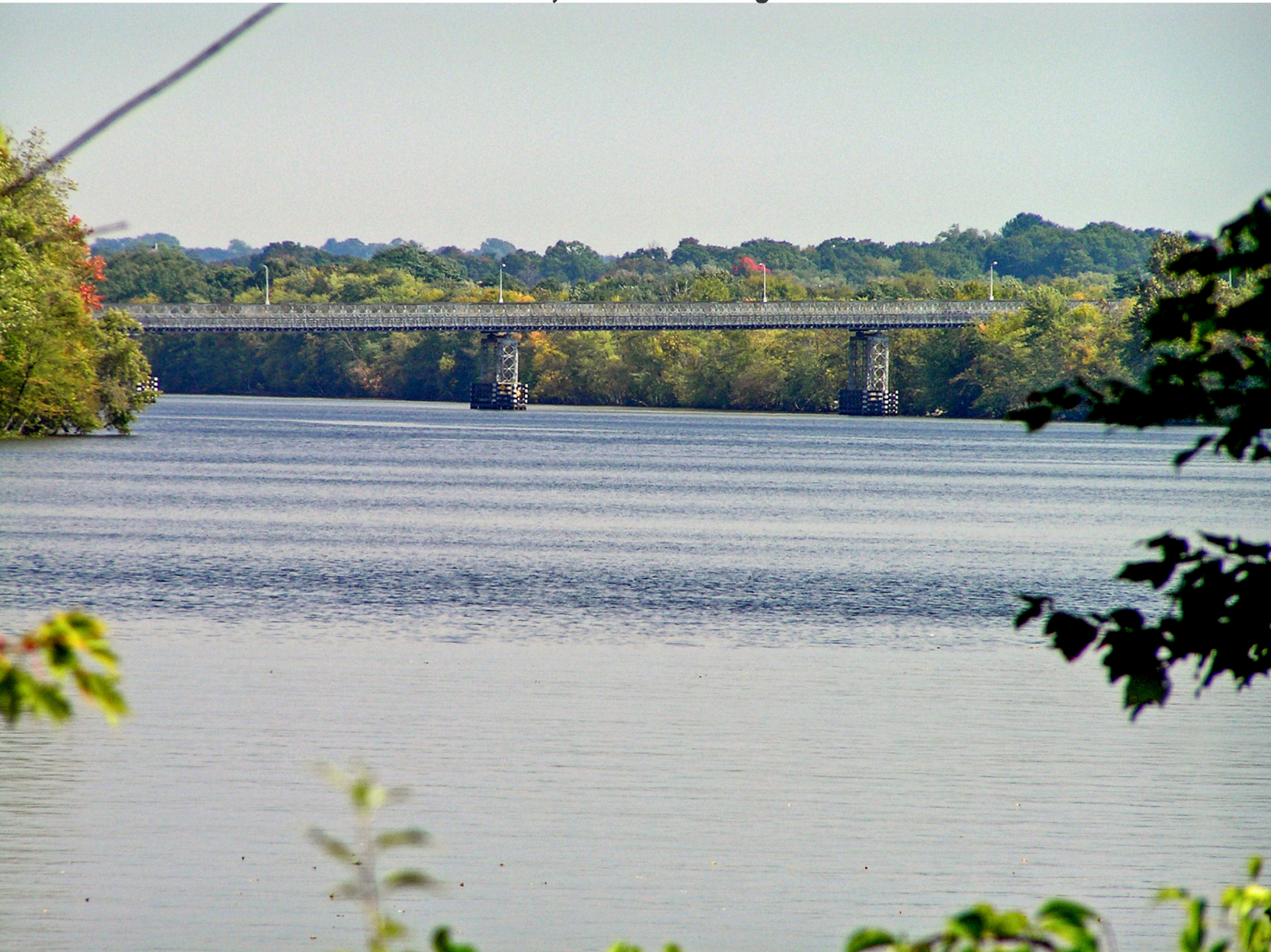
Rourke "Temporary" Bridge Year Built - 1983, Structure Length - 339.2 m
