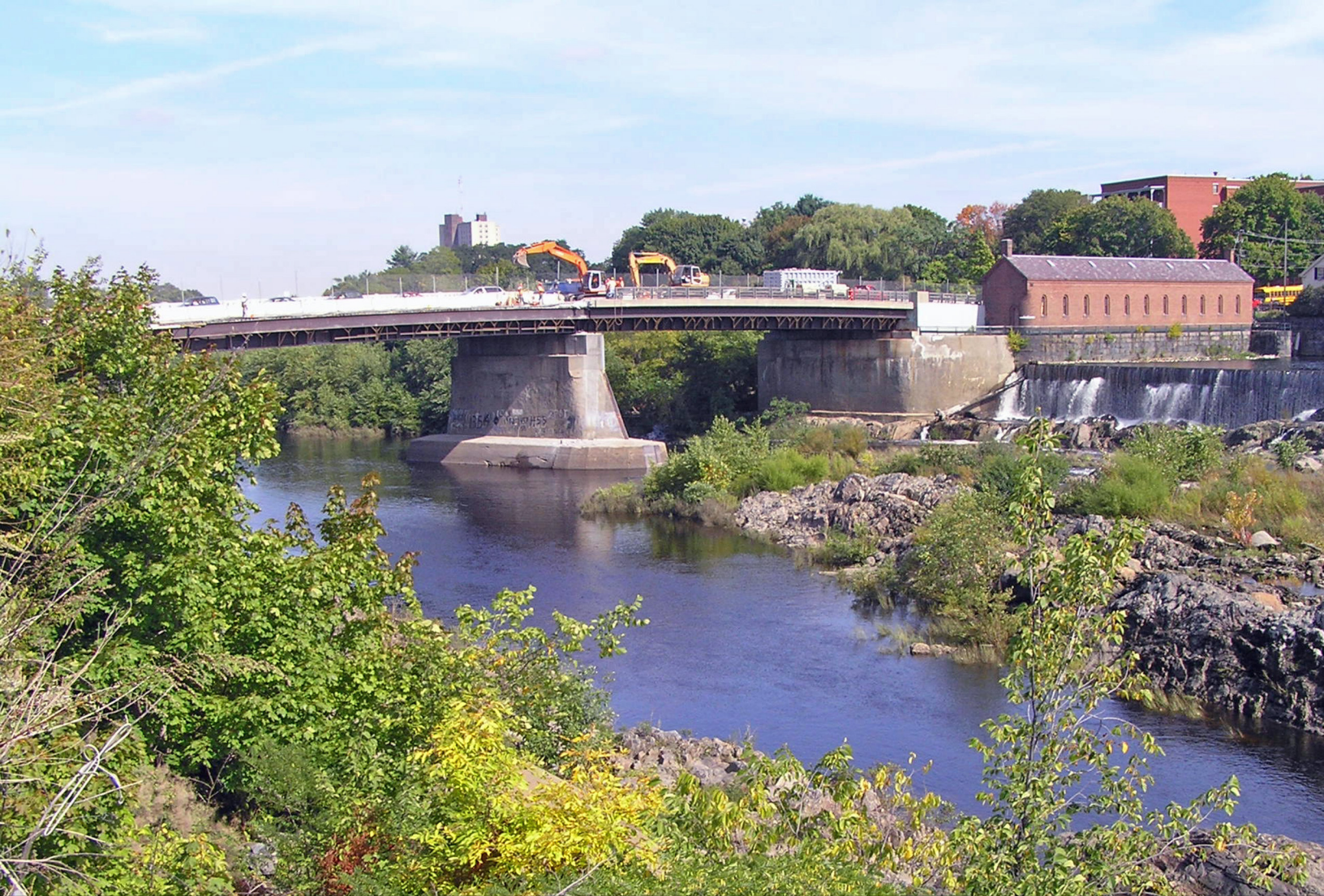
O'Donnell Bridge under reconstruction
