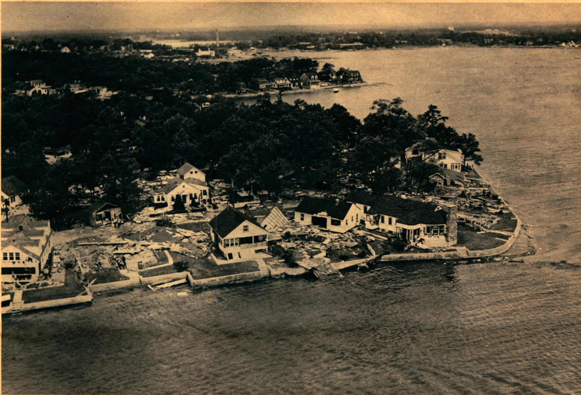
This helicopter photo of the coast at Wareham shows how beach houses, softened by Carol's pounding winds, gave way under tidal waves which roared high over the sea walls. Most severe coastal damage of the storm was centered here and in Buzzards Bay.
