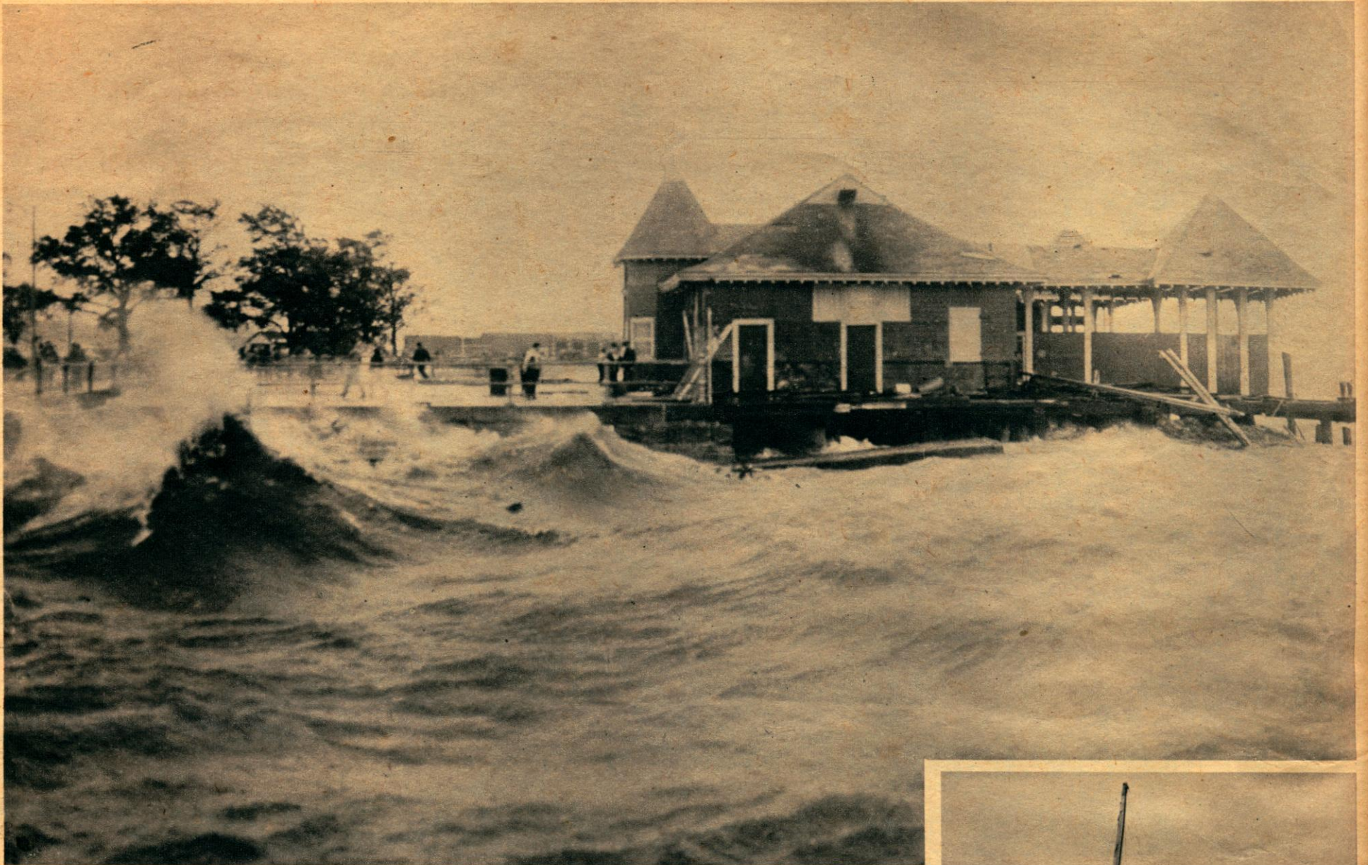
The full power of the hurricane's breakers pounds away at Kelly's Landing, South Boston. Besides splintering the seaward side of the structure, the seas tore away pilings along both sides.
