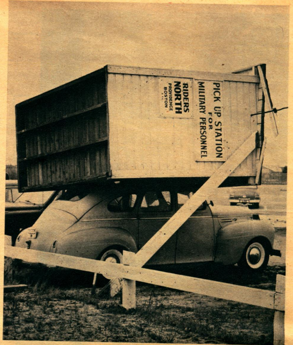
The entire pick-up station was plucked from its foundation and plunked on this car at Quonset Point Naval Station, R. I.
