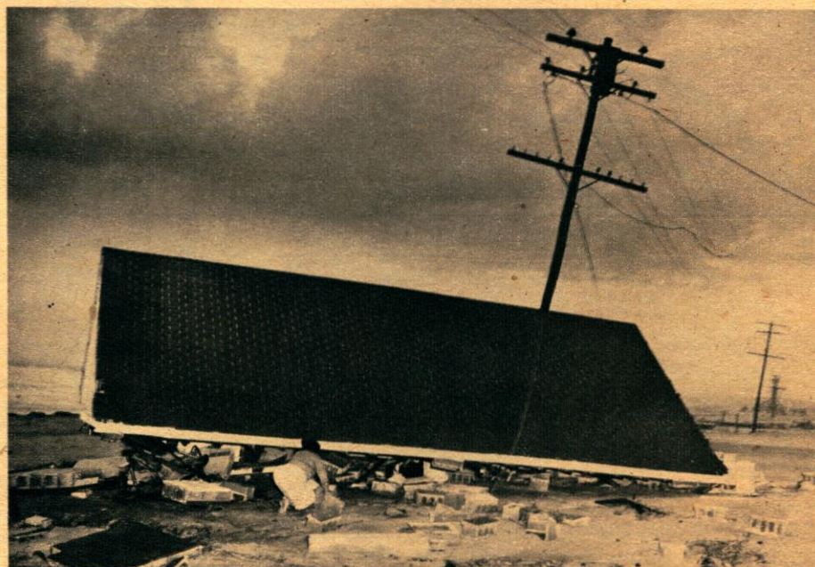
A Westport woman does her best to salvage household articles from beneath the roof of her crushed home. Like most coastal homes, it was abandoned long before the storm sent it crashing.
