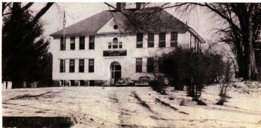
Quessy School 'in West Chelmsford which was closed when the new North school was built.
