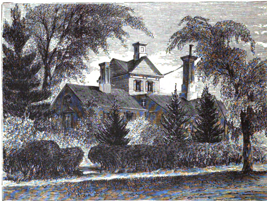
"The Wayside." Hawthorne's Residence.
