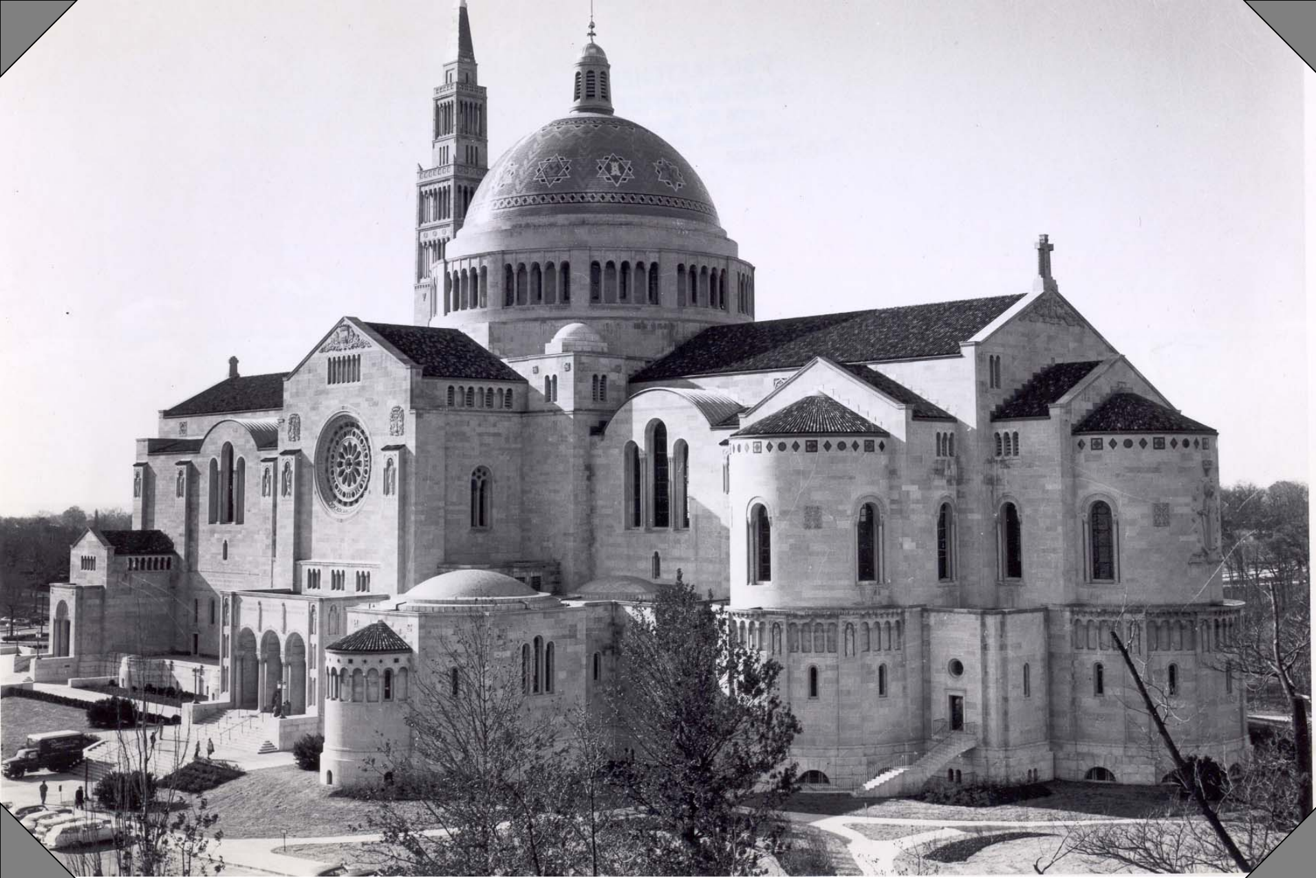
Shrine of the Immaculate Conception, (Michigan Ave. at 4 th St., NE) in Washington, DC was one of the largest projects Fletcher's ever worked on. Begun in 1920, building was stopped due to recession and war and did not resume until 1954. It has both Milford Pink and Chelmsford Grey granite. (See nationalshrine.com )
