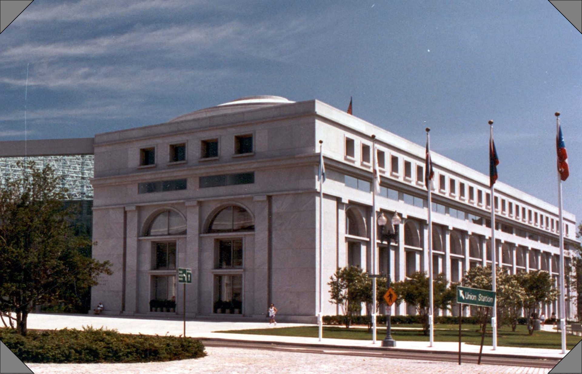
The Federal Judiciary Building in Washington, D.C., completed in 1992, has 65 to 70-thousand cubic feet of Fletcher granite. The stone was fabricated at Westford and Vermont and then trucked to Washington for final assembly. (A Fletcher Photograph)
